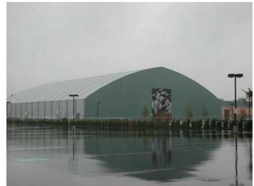
Eagles Indoor Practice Facility NovaCare Complex Philadelphia, PA
