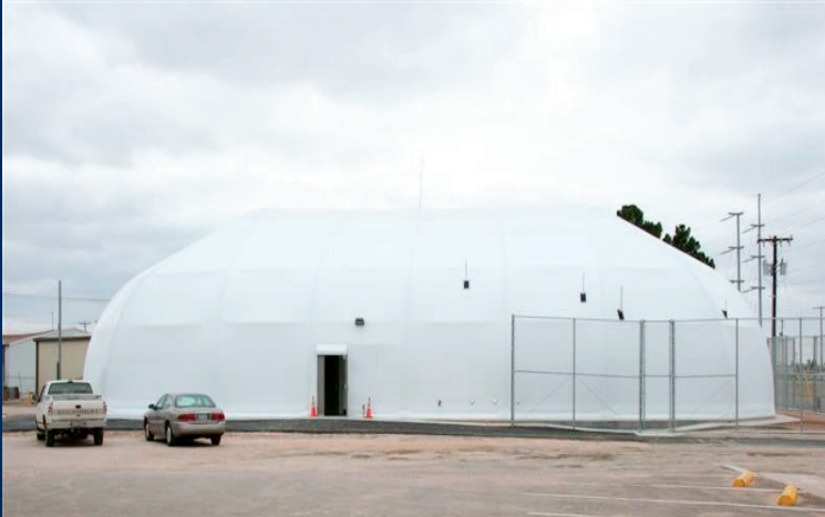
Midland County Correctional Dormitory Midland, Texas
