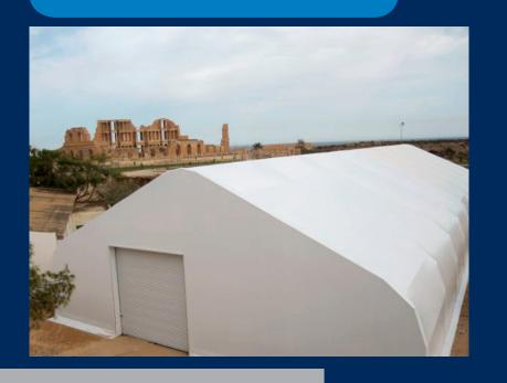
The Hercules Series offers a pre-engineered tension membrane fabric structure that delivers an adaptable, durable, cost effective enclosure.
