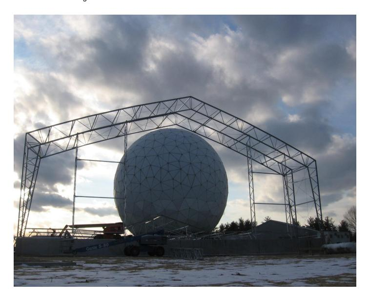
The structure needed to meet interior side wall heights of 34' while meeting all codes for a permanent building. This included a 90 mph wind load and 35 psf ground snow load.
