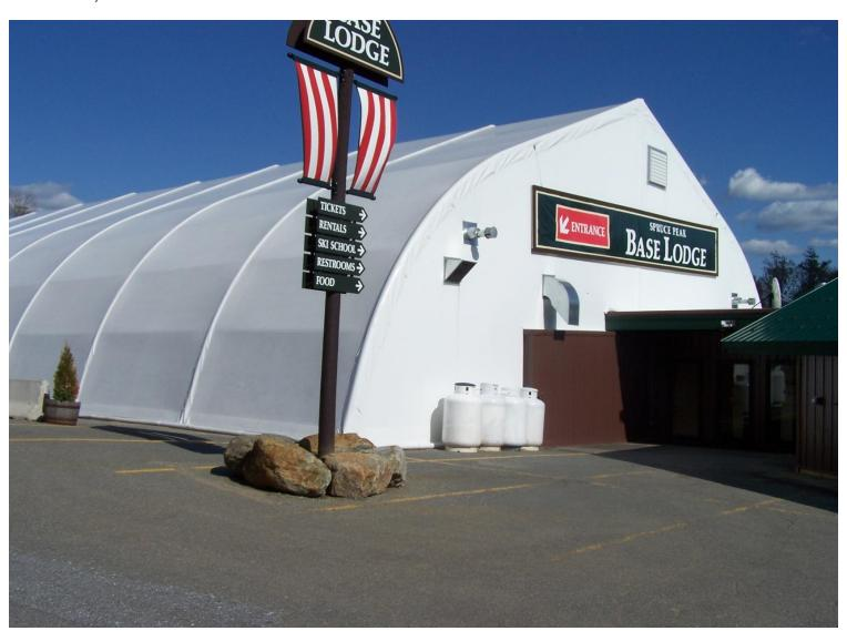
Stowe Mountain Resort was given a customized Tension Fabric System developed to allow for preservation of fabric panels at ground level, giving the customer the ability to relocate structures at a later date without having to require new fabric.
