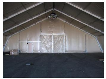
length. Designed initially for U.S. Air Force missions throughout the world, the structure neatly compresses into three slim 8-foot by 8-foot travel containers able to be stored and transported quickly in standard military cabinets. It can be erected and put in use in less than 32 hours by eight untrained workers using no special tools or equipment. It also features heavy-duty 24-oz. Seaman Shelter-Rite<sup>™</sup> tensioned fabric to withstand extreme weather conditions.
