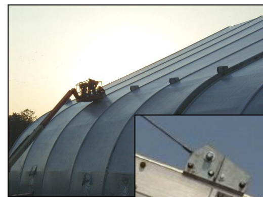
Crane Lift Brackets are installed during initial construction.
