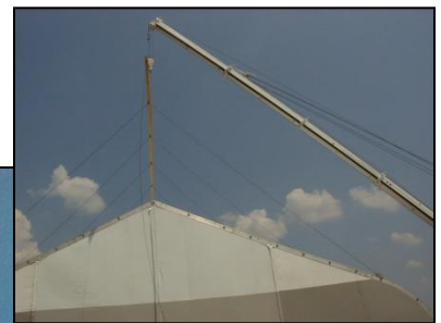
UFS designed Compression Bars to lower costs on crane lifts
