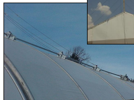
UFS designed Compression Bars to lower costs on crane lifts
