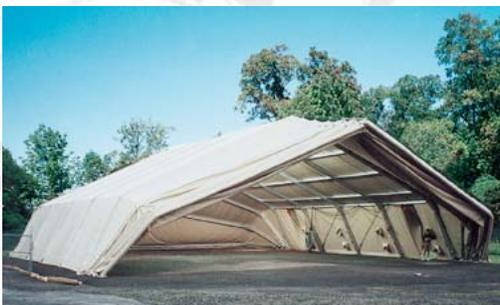
The BBD is a tensile fabric structure, constructed with lightweight aluminum and durable fabric panels. It is available in two widths: 70' and 90' with multiple lengths to accommodate various military uses. The Big Mouth door model is configured on one end with a full-width aircraft/equipment door. Gable ends allow for installation of cargo and personnel door systems. The BBD is designed so
