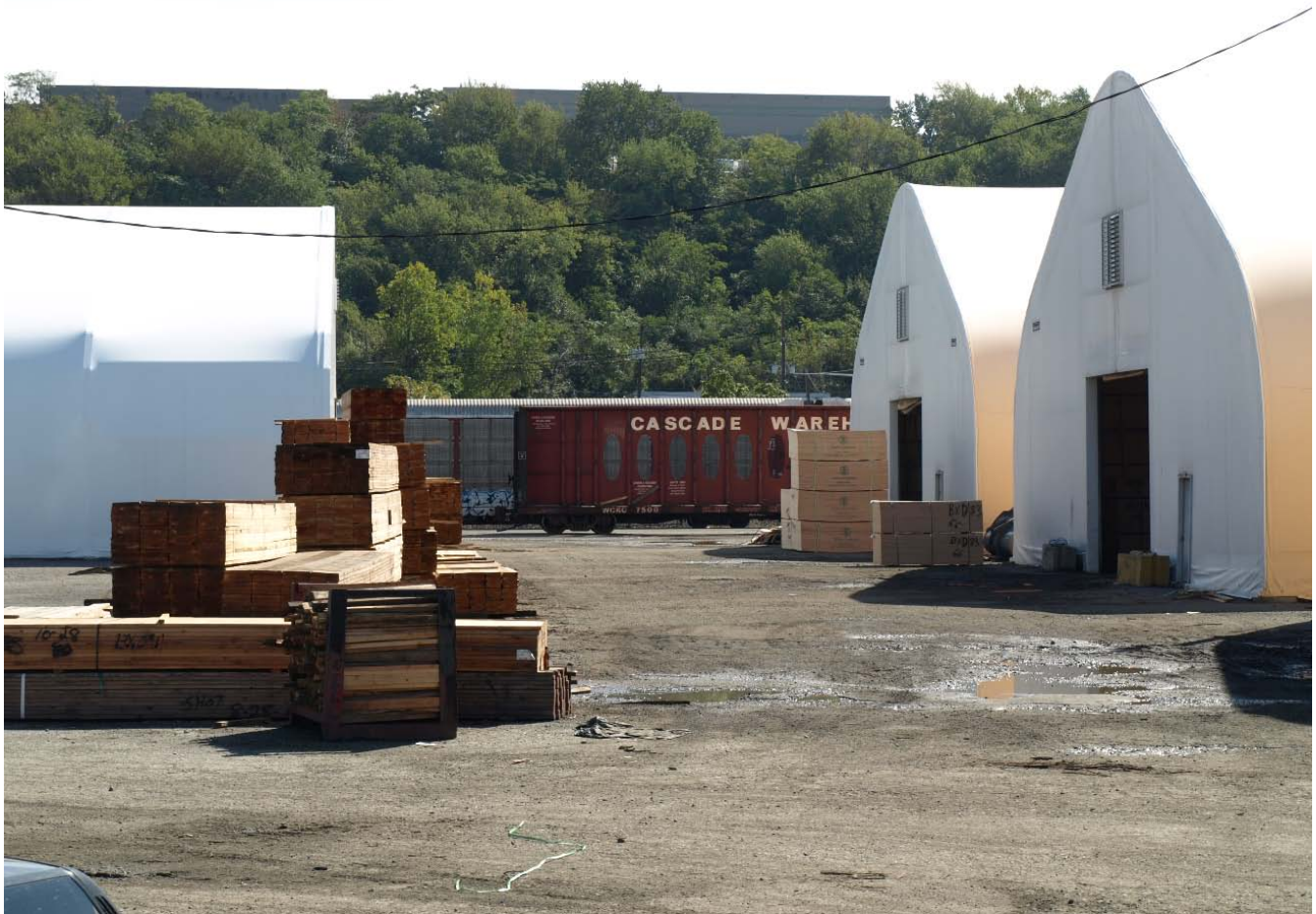
View from the North Bergen, NJ lumber yard entrance. Two of the original Coverall buildings are seen on the right with the new Hercules from Universal Fabric Structures on the left.
