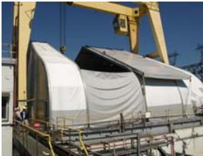
UFS was able to come up with a custom solution that met all of PPL's scope of work. A 92' wide x 64' long, fully customized TFS structure was rented by PPL and designed with a removable bay which allowed the generator to be quickly removed by the overhead crane. The crane
