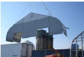
Labor was provided by Universal Fabric Structures and supplemented with labor from PPL, included lifting the portions of the pre-engineered structure with a crane and then mounting onto a raised concrete deck platform. Paul Frazza, Generation Services Engineer for PPL Corporation was impressed with the overall performance of the structure, "Overall, UFS presented us with a creative approach to accommodate our crane use within the building."
