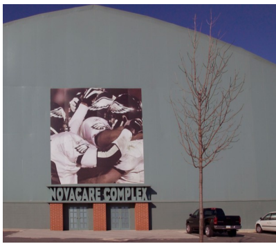
The Eagles Novacare practice facility is a Universal Fabric Structure
